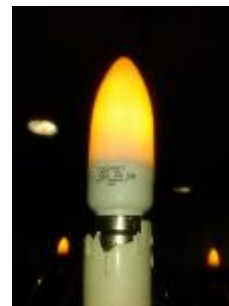
Figure 5. Retrofitted more efficient LED lighting
